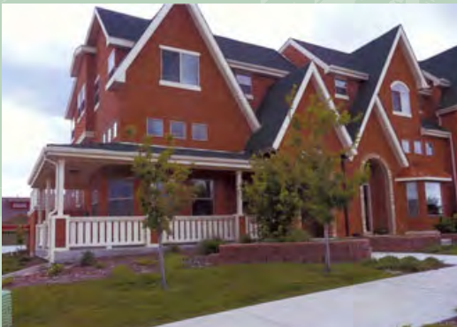
Loan value: $800,000 Seven entry level town homes in desirable Parker, CO Vertical spec construction financing 50% loan-to-value
